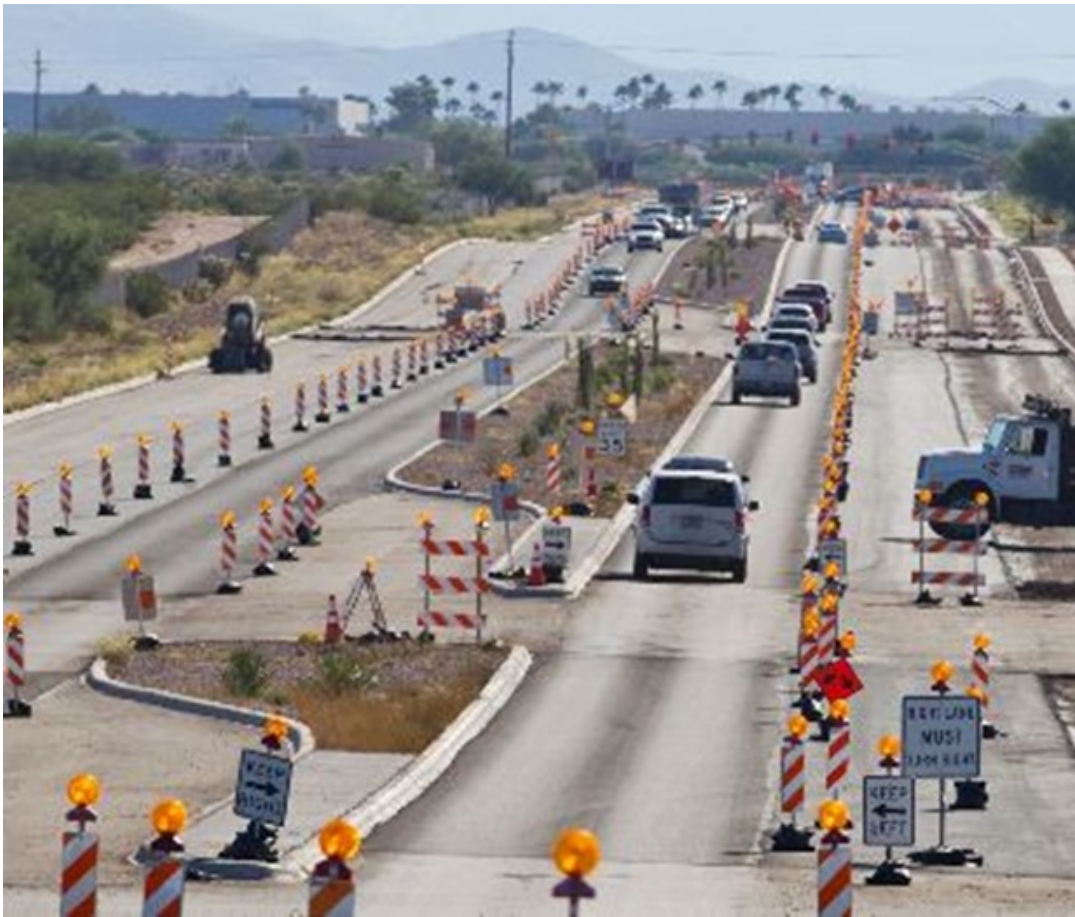
A historical look at Green Valley roadwork by Pima County in 2018.
